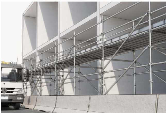
Figure 36: Use of concrete barriers around scaffold in a trafficable area
