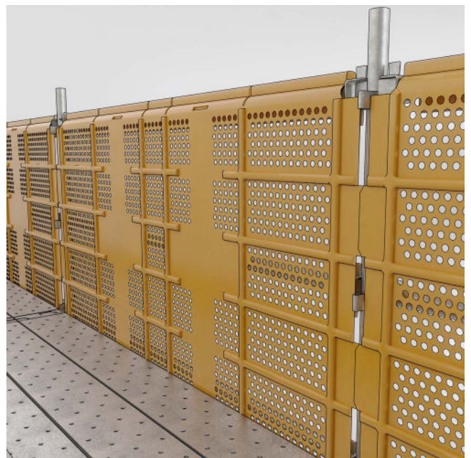
Figure 35: Use of perimeter containment screens, shade cloth and brick guards to contain falling objects
